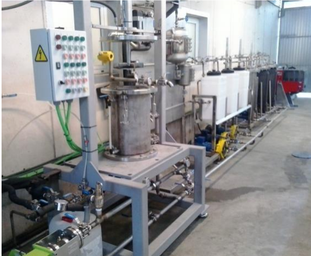
Reactor 2 Installation Overview
